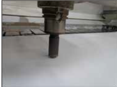
Wet drilling using a Drill Bit
